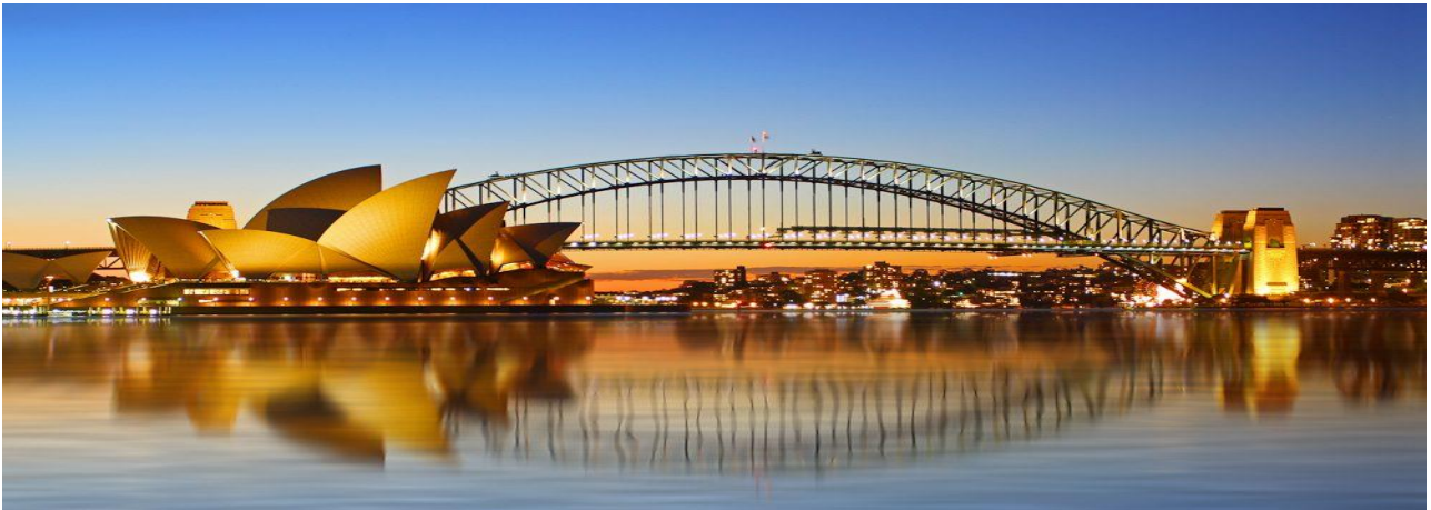
Sydney Harbour Bridge
