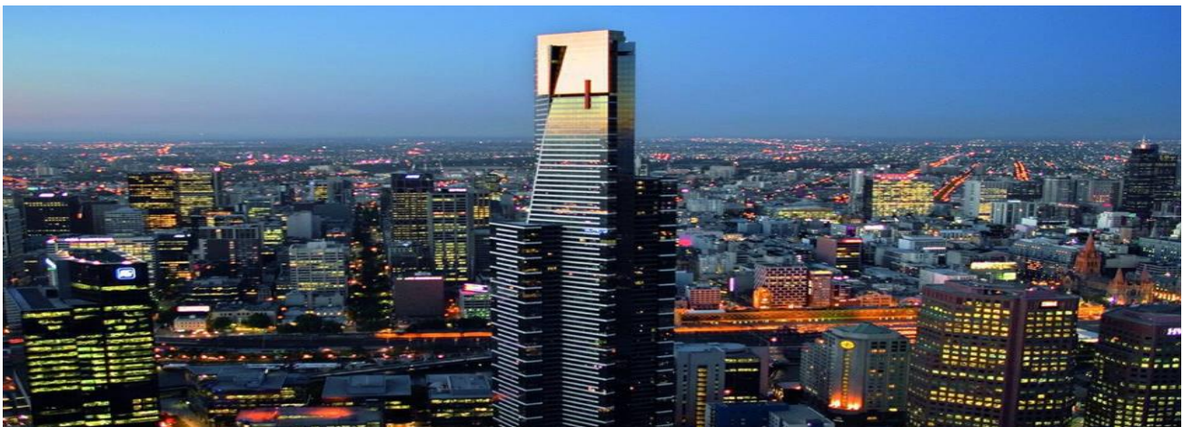
Modern skyscrapers on Collins Street.
